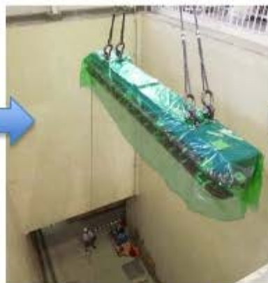
move into tunnel
