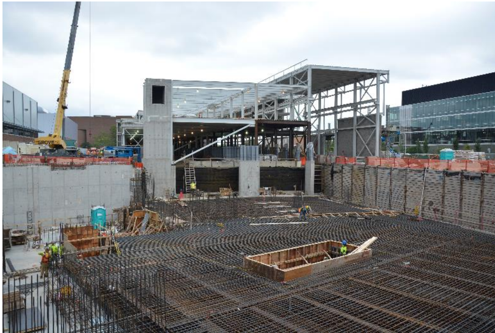
View of tunnel lid re-steel looking east
