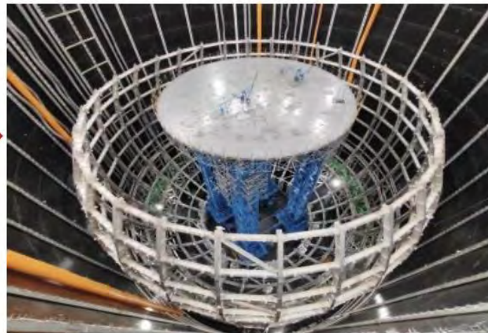
Platform for Acrylic assembly
