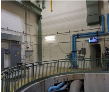
MINOS access shaft
