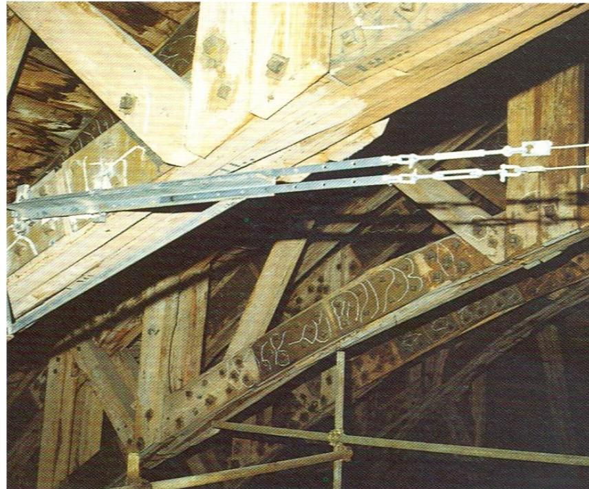
Sensors consisted in a couple of wires of invar (nickel-iron alloy) and steel to compensate for thermic variations
